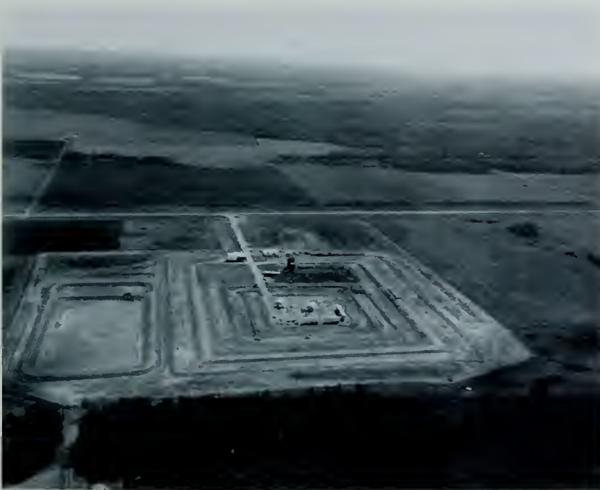
Fig. 2-36. Four remote SPRINT launch sites equipped with 12-16 SPRINT launch stations provided additional protection.
